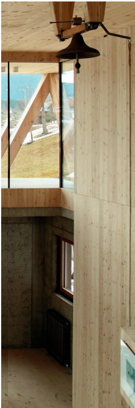
1 Das Atelier reicht vom Sockel- geschoß ins Erdgeschoß The art- ist's studio rises up from the con- crete plinth to ground floor
